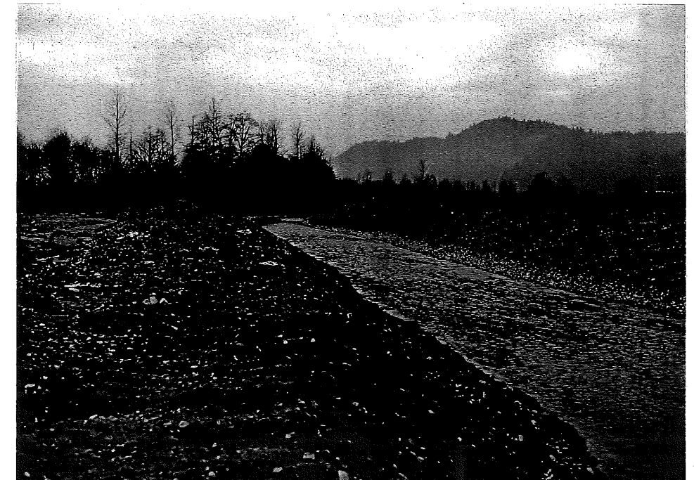
Photo 4. View downstream from below Farms Road bridge showing spoil piles along channel.
